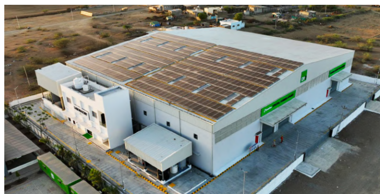
SOLAR PANEL INSTALLATION AT CR3 INDIA
