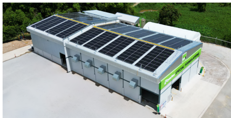
SOLAR PANEL INSTALLATION AT CR3 THAILAND
