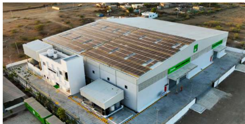
SOLAR PANEL INSTALLATION AT CR3 INDIA
