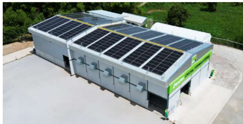
SOLAR PANEL INSTALLATION AT CR3 THAILAND
